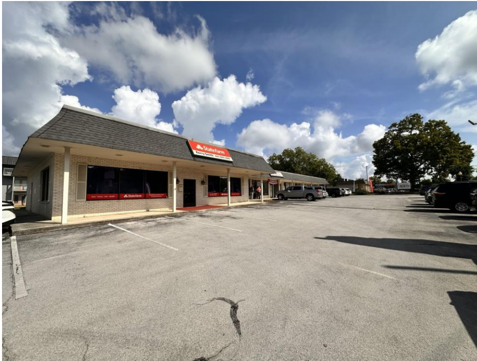
Street-front elevation along Dayton Boulevard
